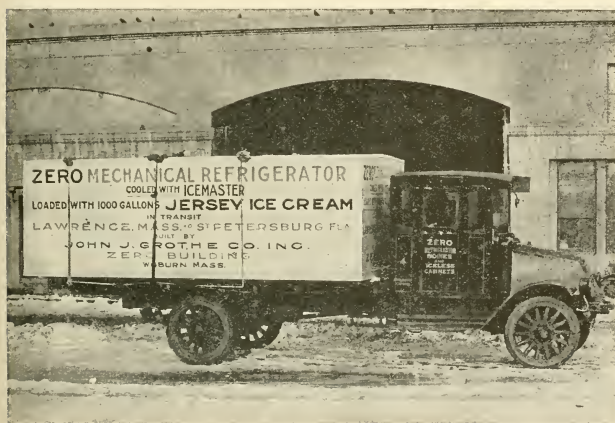
FIG. 182.—CORKBOARD INSULATED LONG-DISTANCE REFRIGERATED ICE CREAM TRUCK.
