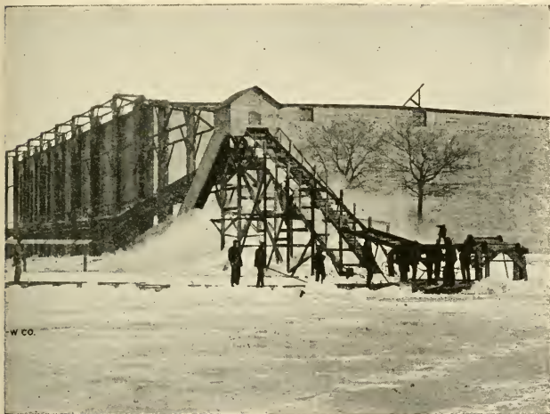
FIG. 150.—SAWDUST INSULATED NATURAL ICE HOUSE.
