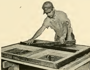
FIG. 164.—CABINETMAKER PLACING CORKBOARD IN STILES AND RAILS BETWEEN DOOR OPENINGS.
