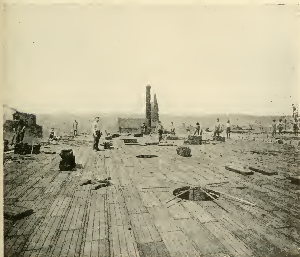
FIG. 131.—PLACING FIRST LAYER CORKBOARD IN CEILING FORMS BEFORE CONCRETE IS Poured.
