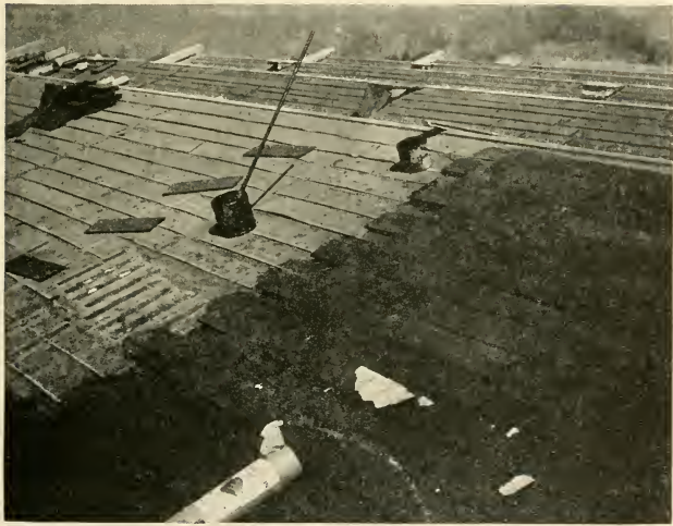
FIG. 22.—CORKBOARD INSULATION BEING APPLIED TO SAW-TOOTH ROOF CONSTRUCTION.
