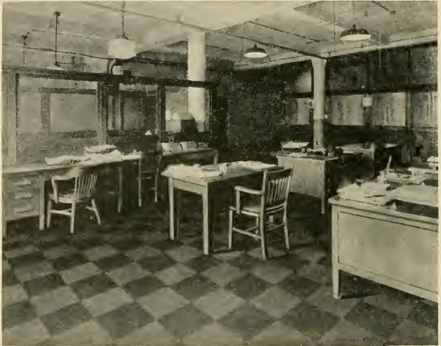
FIG. 21.—CORK TILE FLOOR IN MODERN OFFICE.
