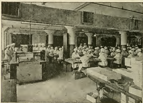
FIG. 66.—CORKBOARD INSULATED CHOCOLATE DIPPING ROOM WITH COLD AIR DUCT CIRCULATING SYSTEM.
